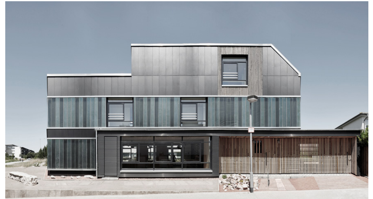
... and reused for the cladding of a (90% recycled) home.
